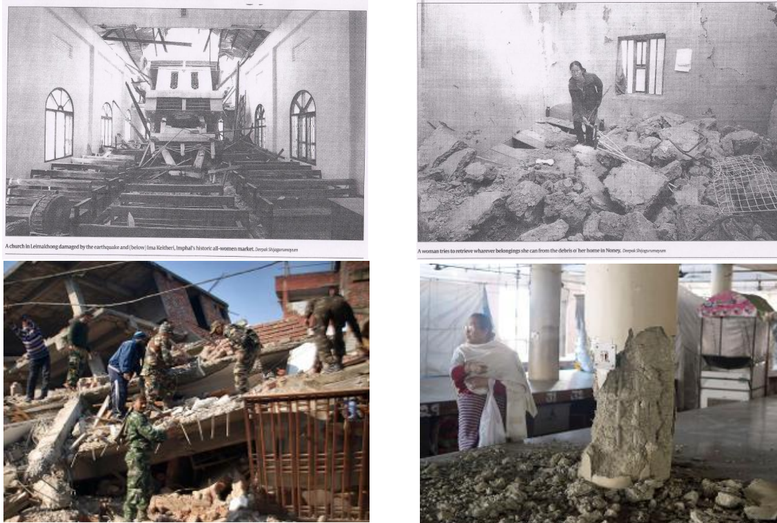
Fig. 5a: Clockwise from top (a) Damaged Imphal church (b) Collapsed house in Imphal (c) Collapsed new buildings in Imphal market (d) Collapsed walls and failed pillars in All Women Market
